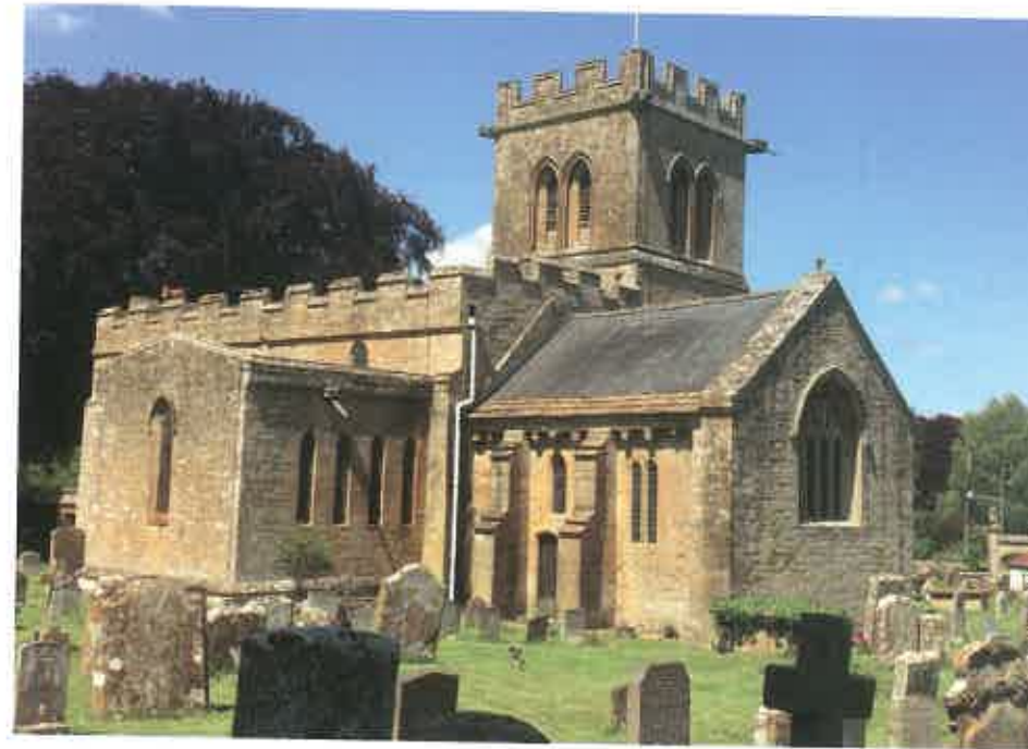
► St Mary's Church, Stoke-sub-Hamdon, Somerset
