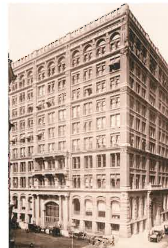
▼ A photograph of Chicago's Home Insurance Building shortly after it opened in 1884. This was the world's first skyscraper
